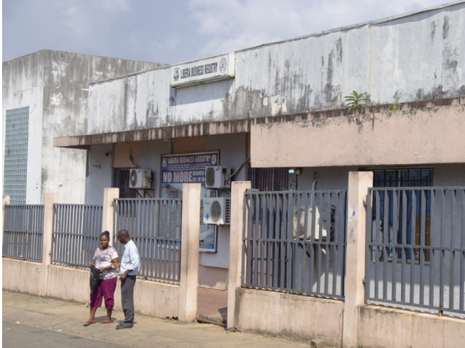
Liberia's domestic business registry, near Broad Street, Monrovia. The domestic registry services Liberian companies and looks run down compared to LISCR's shiny offices.
